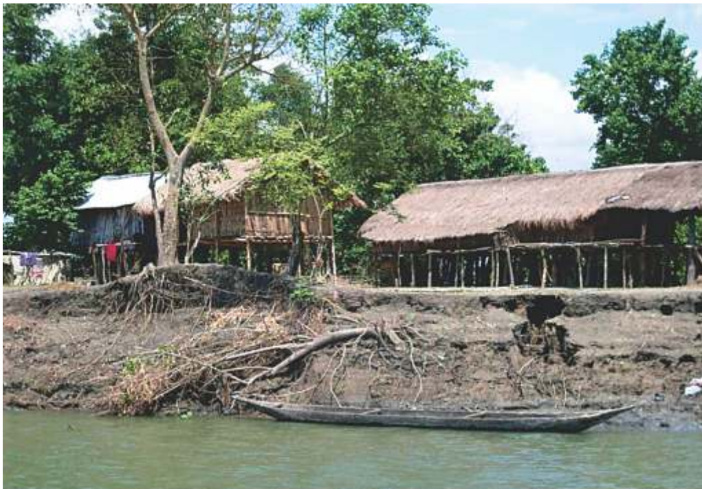
A Mising tribe village in upper Assam's Lakhimpur district with houses built on stilts to escape the wrath of floods. The houses are designed with vernacular, traditional technology.
